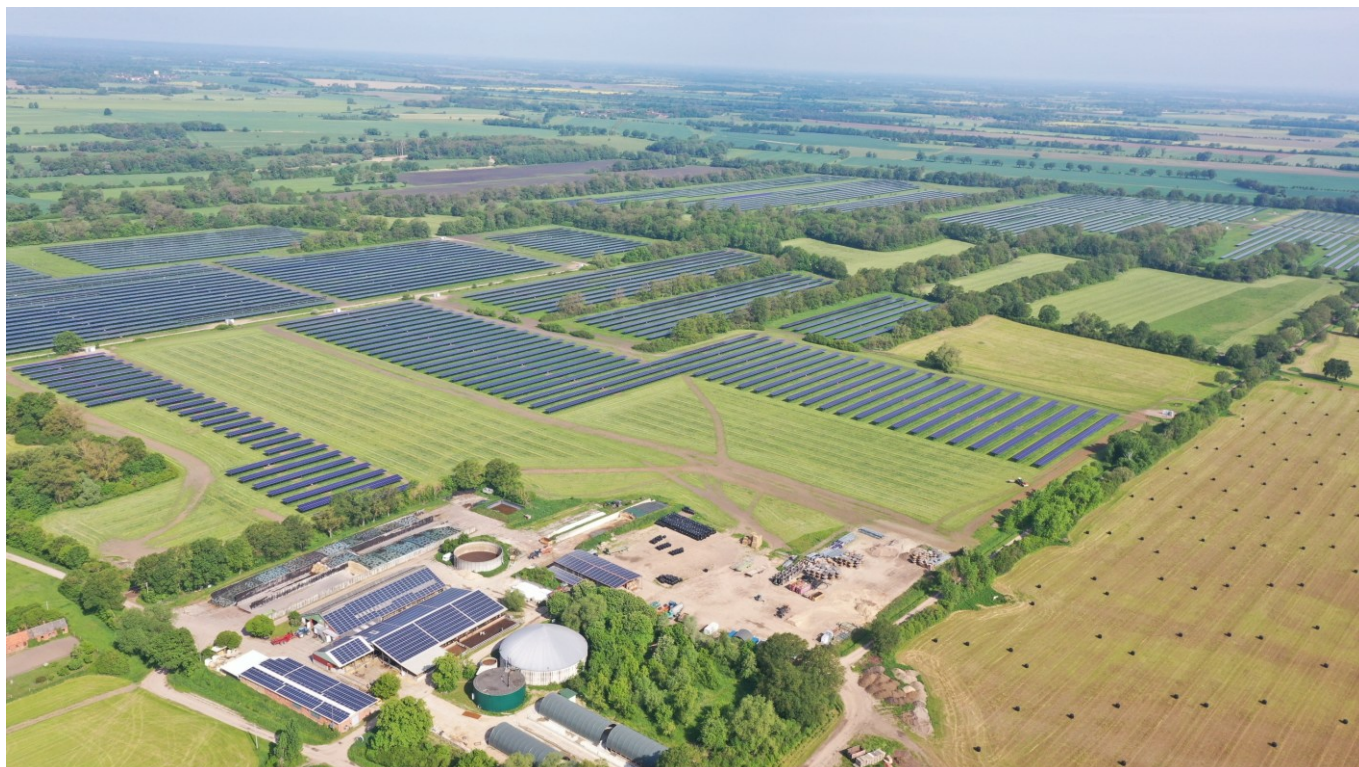
The 69 MWp Agri-PV park in Schwarzhof, Saxony-Anhalt. Photo credit: FEFA Projekt GmbH.
